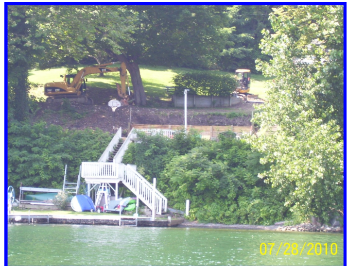
Construction of retaining wall at lakefront home. Project has been completed.
