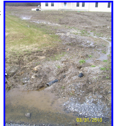
Picture shows area of failing septic system and its proximity to the roadside ditch from the 9/21/2009 investigation. Septic system was repaired in 2010.
