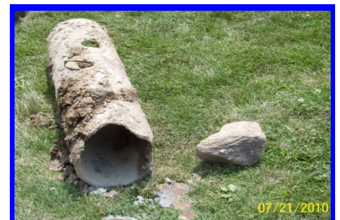
Picture shows rock that had broken through sewer line, as well as two other holes in the section of line.
