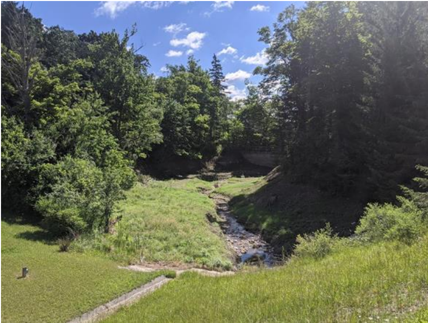
2: Sediment Retention Basin - After Seeding
